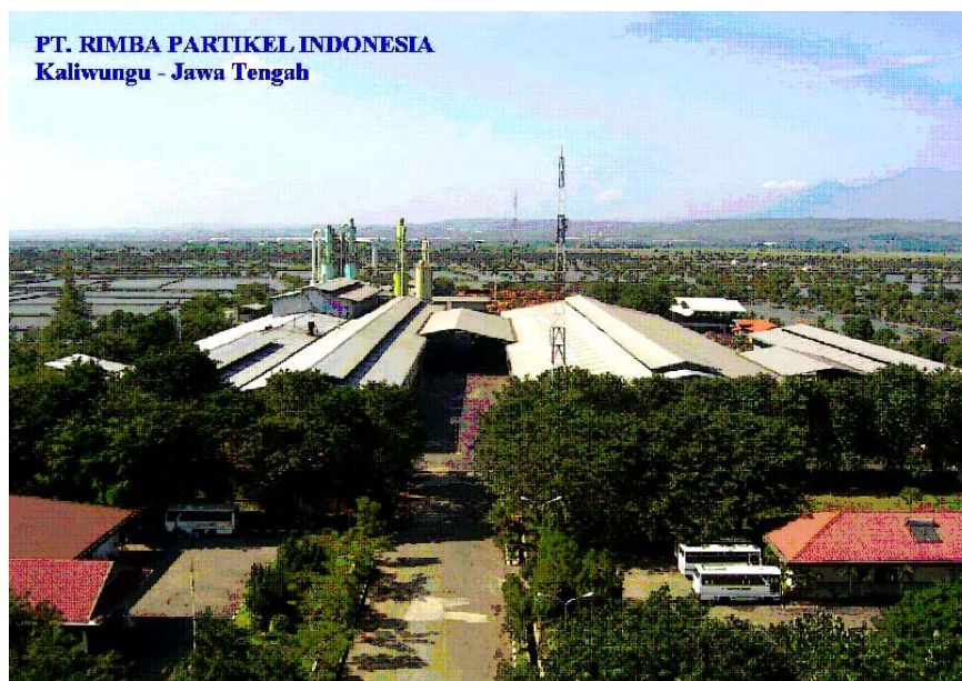
Fig-1: Full view of the plant
