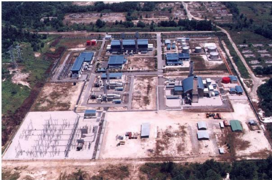
Aerial view of Bintulu Power Station and Combine-cycle Project Location
